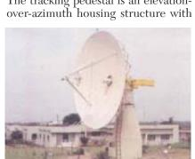
📤 Fig. 8 Dual-band, single-channel monopulse tracking-feed antenna.
